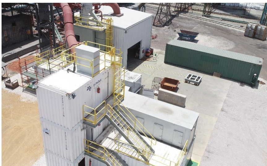
DST GlassLock Facility in Namibia
