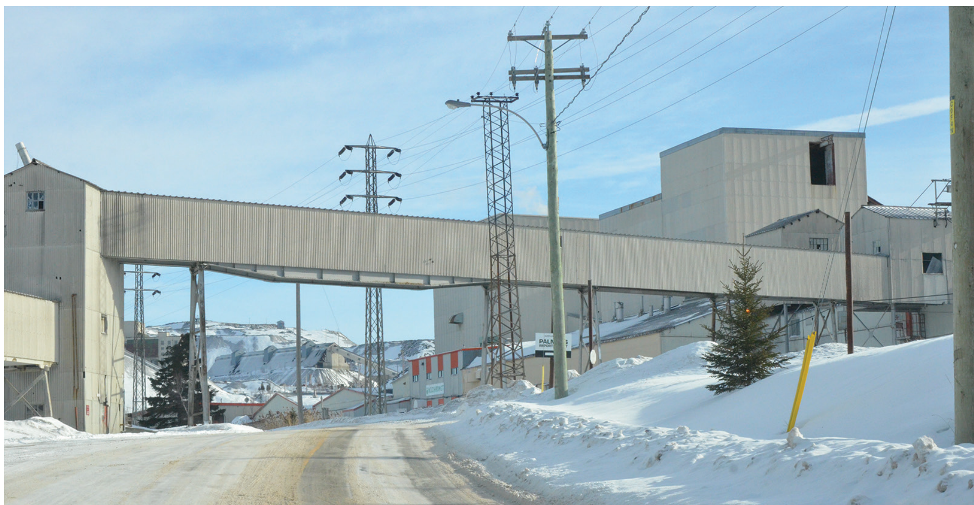
Dundee Sustainable Technologies' Clevr plant and technical facilities in Thetford Mines, Que. DUNDEE SUSTAINABLE TECHNOLOGIES
