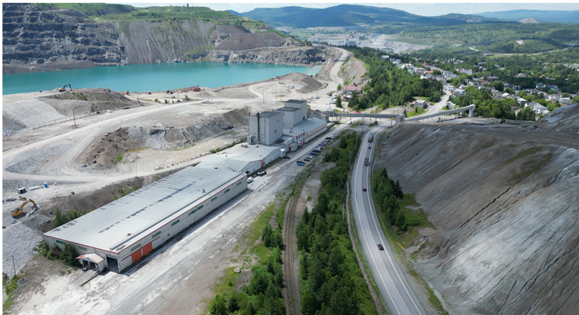
DST's Plant & Technical Facilities in Thetford Mines, Canada
